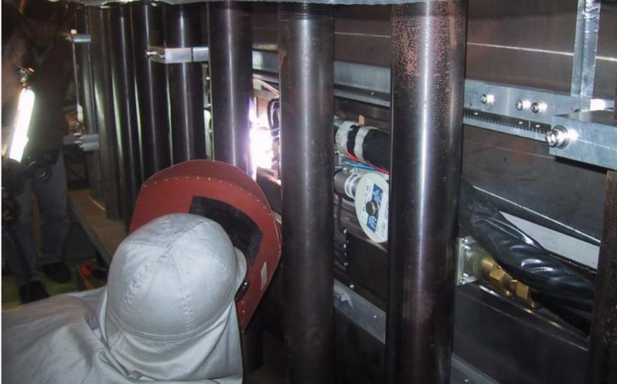
Longitudinal shell welding by two automatic welding machines.
