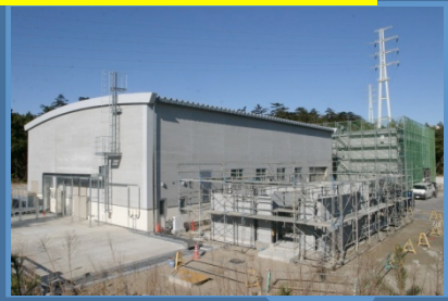
Neutrino monitor building
